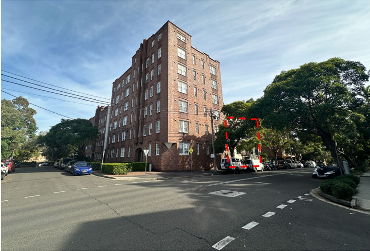
looking south-west from the Liverpool Street and Darley Street intersection
