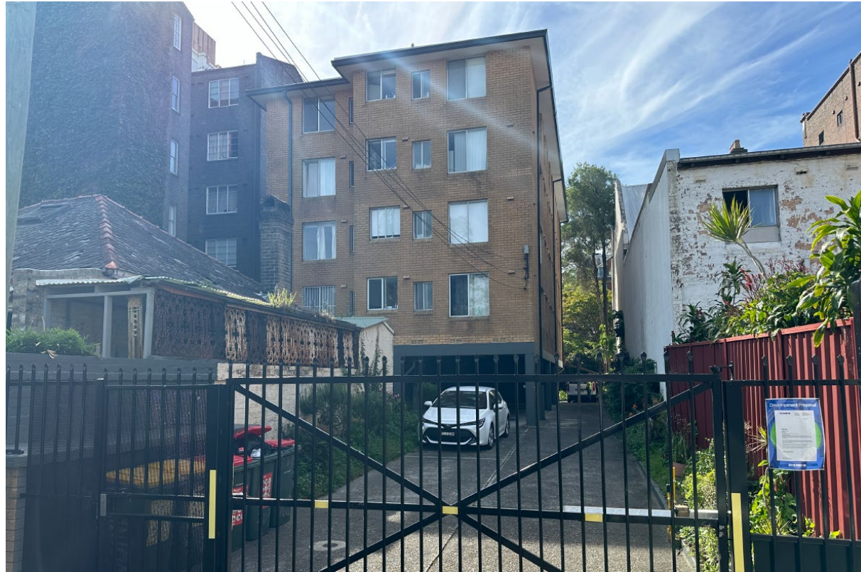
Looking north towards the rear setback of 349 Liverpool Street and the heritage item cottage of 1 Darley Place to the left
