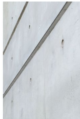
OFF FORM CONCRETE
